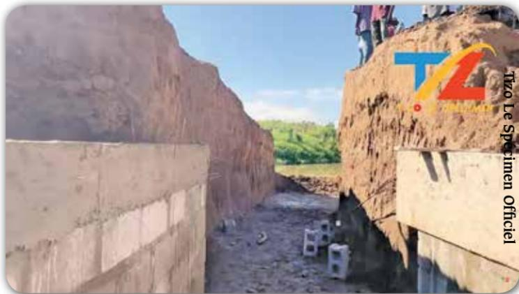
A video filmed on Sep. 10, 2023 shows that the canal has only a few more meters to be built before it is connected with the Massacre River.
